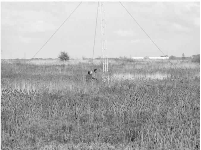
Jack VE3WBT & Jim VE3EEZ repairing the 160 m loop
