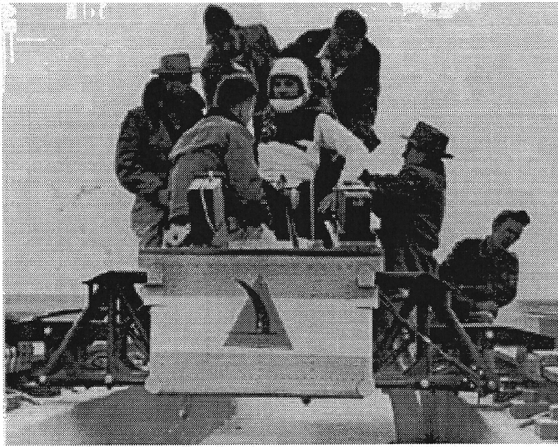
The picture shows Dr John Paul Stapp strapped aboard a sled in an experiment testing the effects of sudden deceleration.
