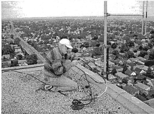
John Servicing the VE3NCF Antenna
